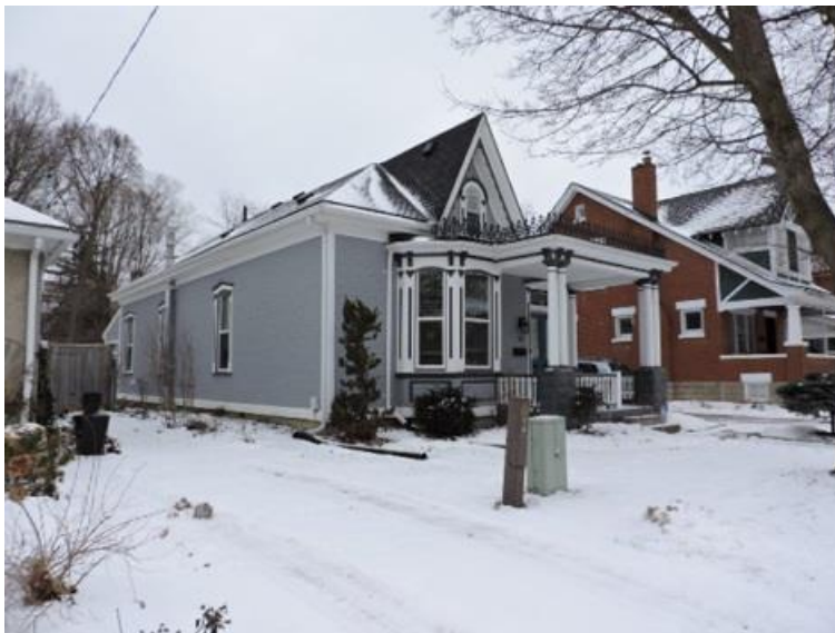
Photo 2: West elevation of 68 Bruce Street (AB, 2016)
