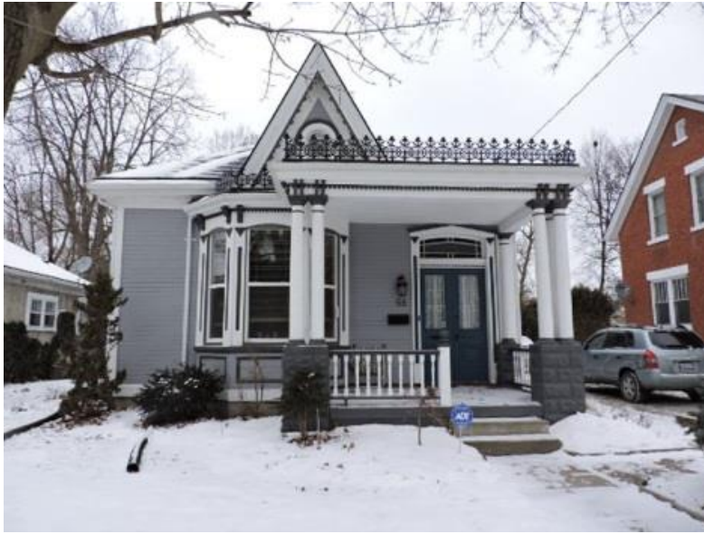
Photo 1: Front façade of 68 Bruce Street (AB, 2016)
