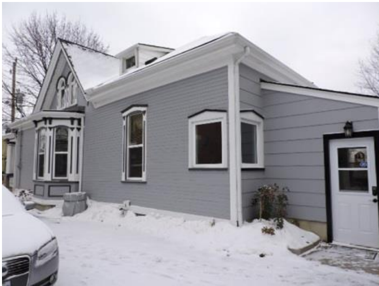
Photo 4: Rear of east elevation of 68 Bruce Street (AB, 2016)
