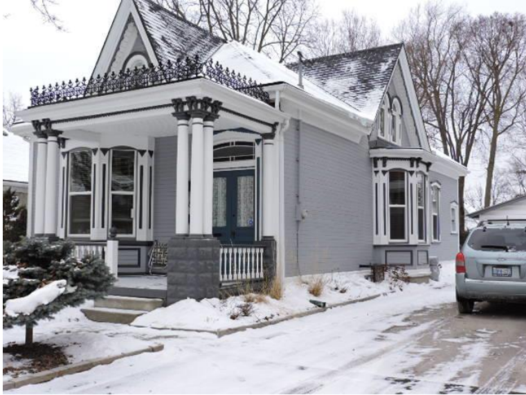
Photo 3: East elevation of 68 Bruce Street (AB, 2016)
