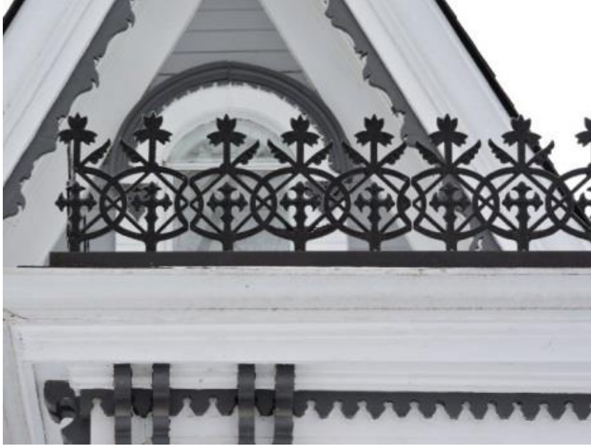
Photo 11: Detail of wrought iron cresting, bargeboard trim, and gable window (AB, 2016).
