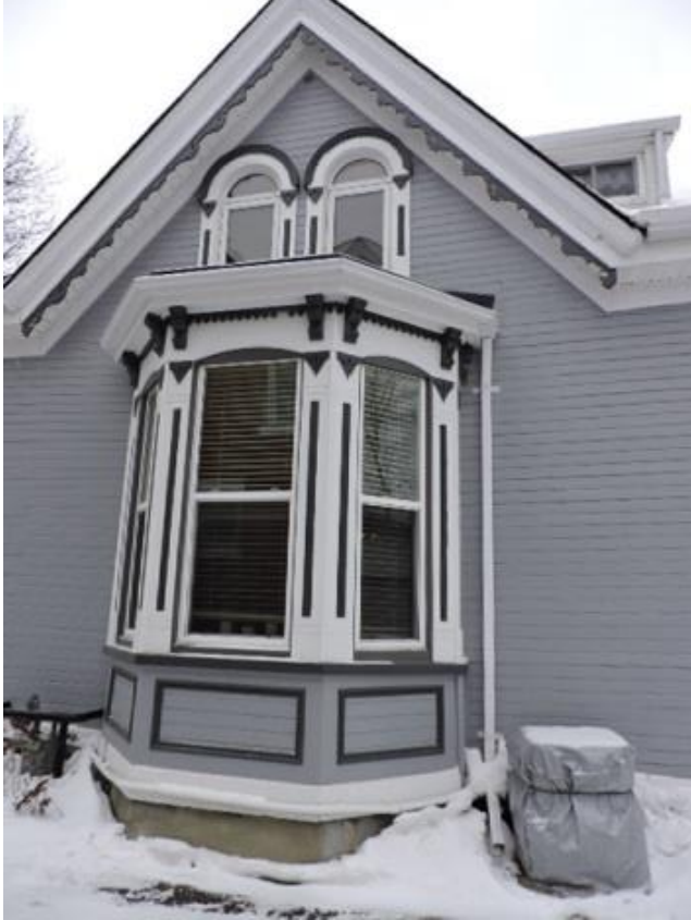
Photo 5: East elevation bay window (AB, 2016)
