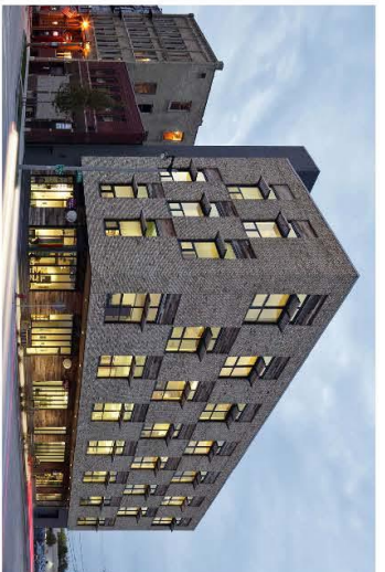
Example of contemporary 4 storey mixed-use development lining up floor heights and horizontal datum lines.
