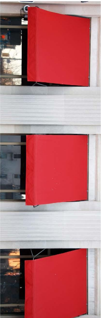
Awnings installed in Downtown London, ON
