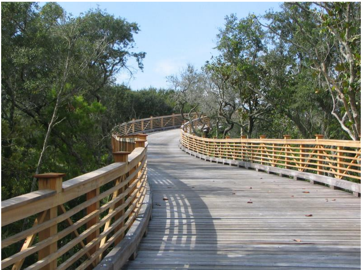
Figure 1 A pedestrian bridge that utilizes natural materials. Source: Nature Bridges http://www.naturebridges.com/gallery_new/golf_cart.php#prettyPhoto
