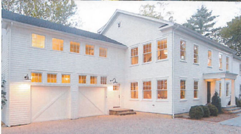
EXTERIOR SIDING DETAIL OF HOME
