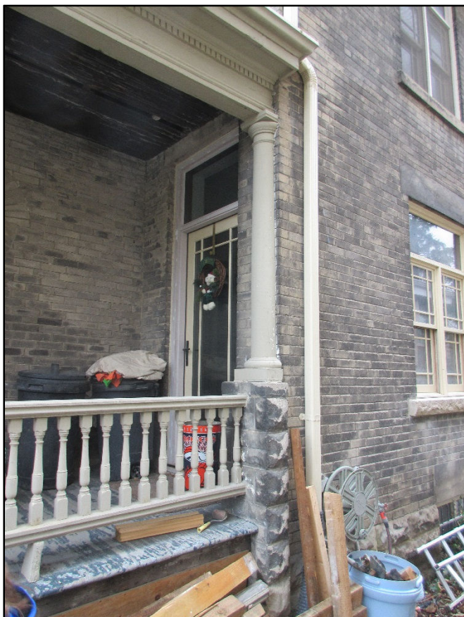
Image 2: Detail of porch (prior to alteration).
