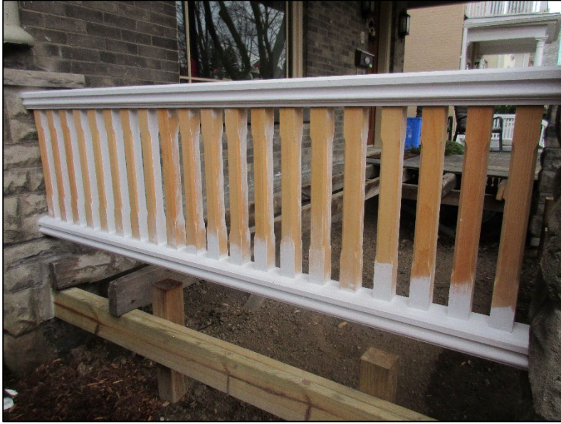
Image 3: Detail of porch (showing replacement spindles).
