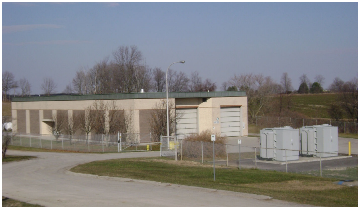
Exterior of the Arva Pumping Station
