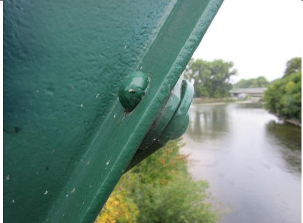
Image 12: Detail of the pin-connection of the King Street Bridge (September 29, 2015).
