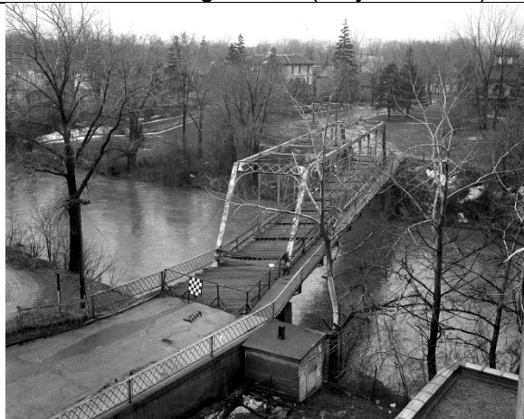
Image 4: Image of the King Street Bridge, with the cantilever sidewalk to the north. Note the barrier preventing access across the King Street Bridge (courtesy of the London Free Press , October 3, 1957).
