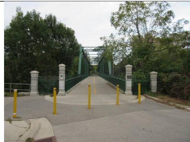
Image 13: West approach to the King Street Bridge (September 29, 2015).
