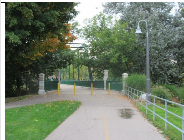
Image 9: East approach to the King Street Bridge (September 28, 2015).
