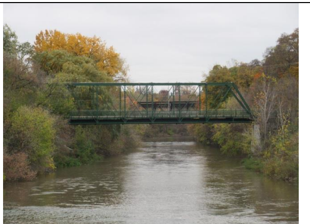
Image 16: King Street Bridge seen from Mitchell A. Baran Park (October 28, 2015).
