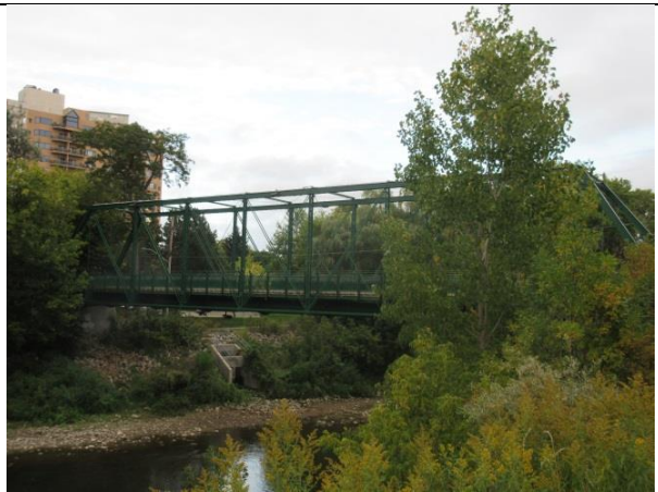
Image 14: View of the King Street Bridge from the northwest (September 29, 2015).
