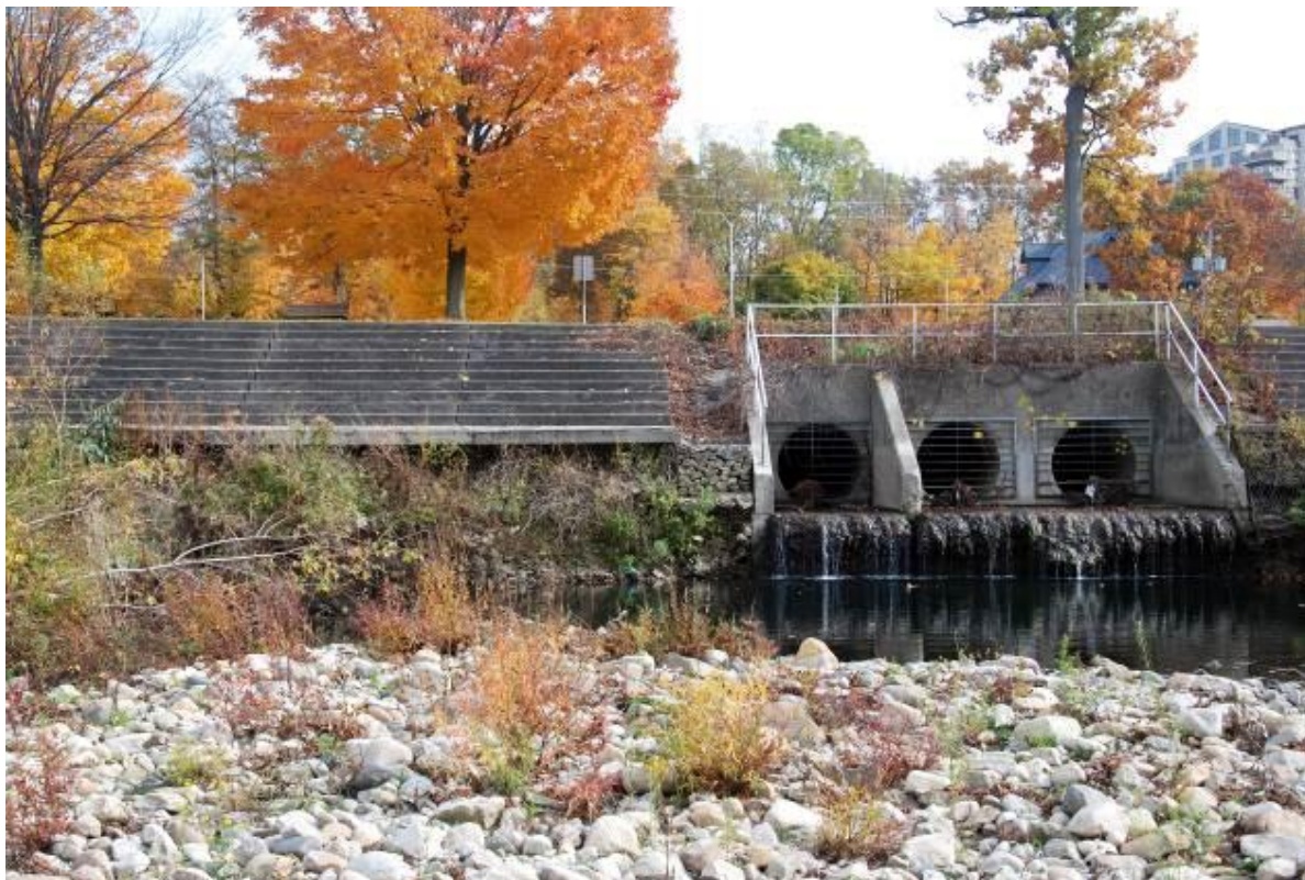
Photo #5: Storm Sewer outfall & bleachers at Rowing Club
