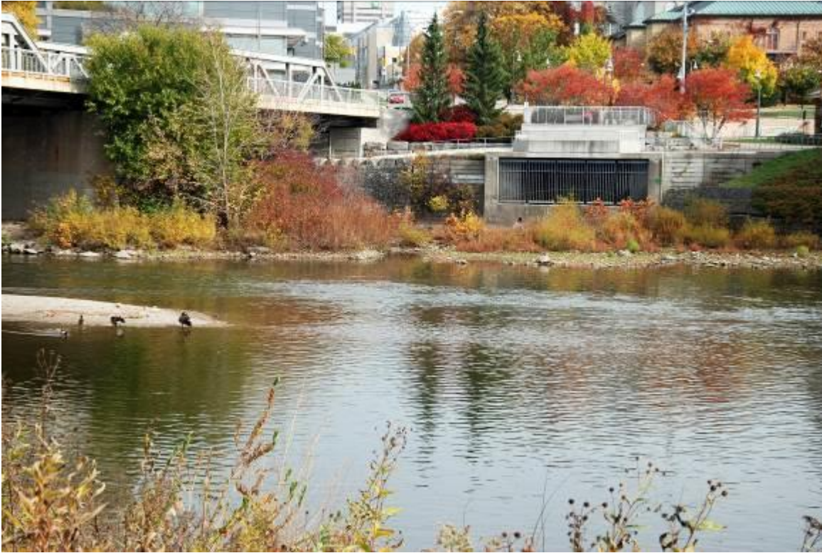
Photo #3: Storm Sewer outfall at the Forks
