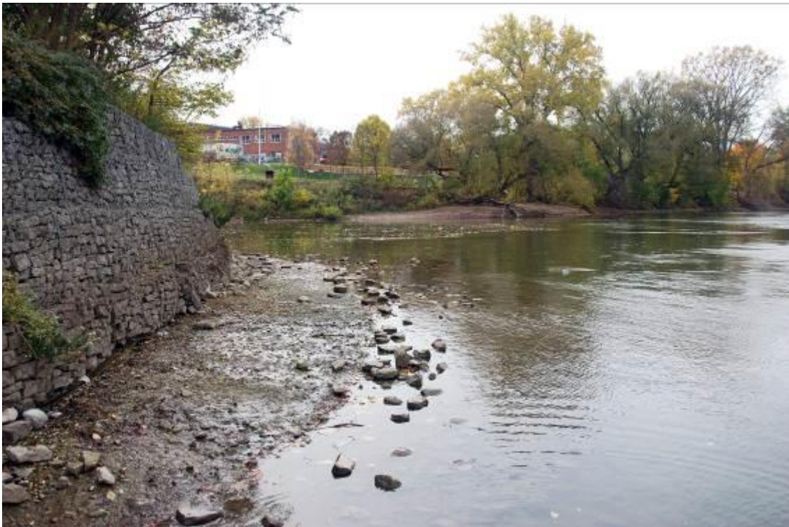
Photo #2: Gabion basket wall at the Forks
