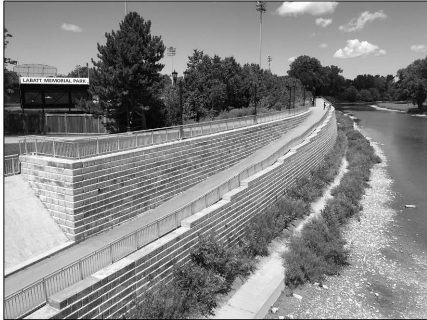
Figure 1 Phase 1 of West London Dyke Replacement.
