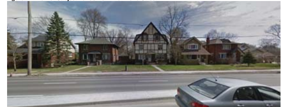
Figure 3 – View of subject lands from Raymond Avenue
