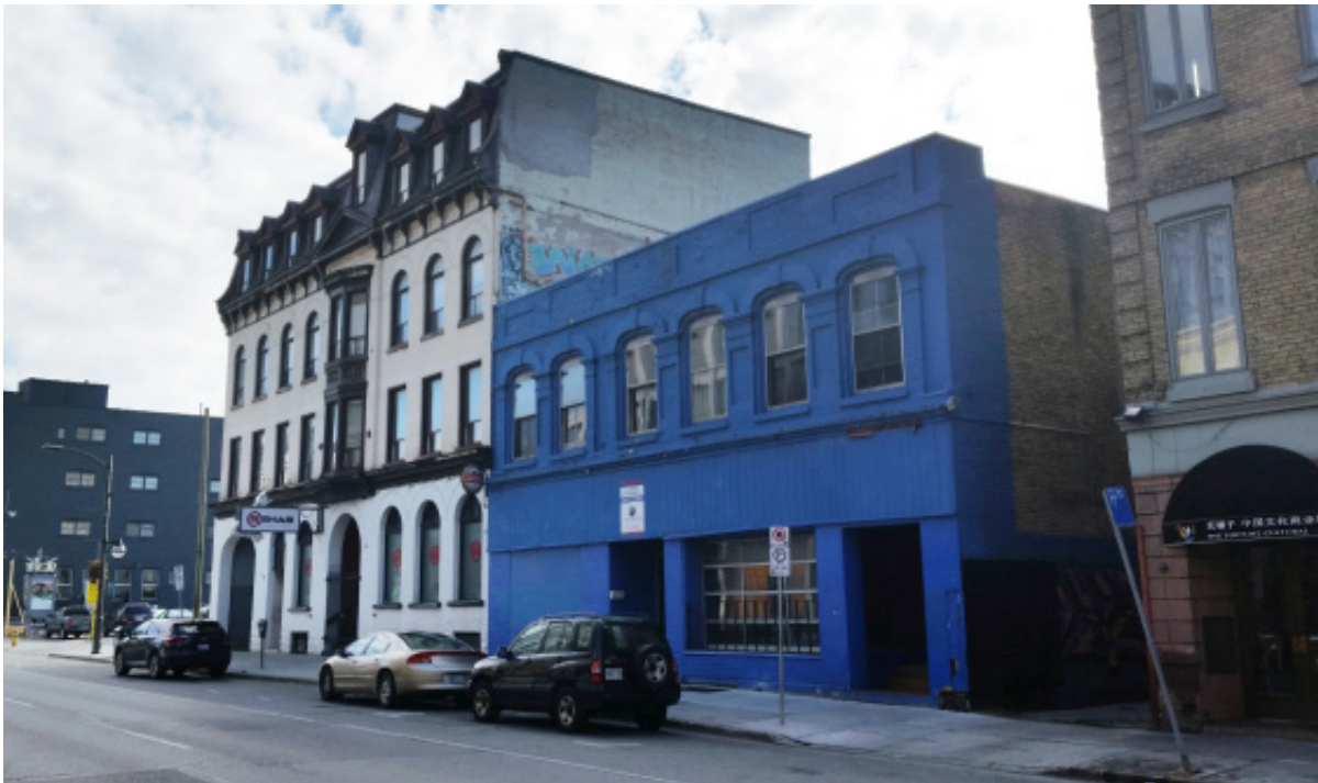
21. Contextual view from the west (Source: ERA Architects)
