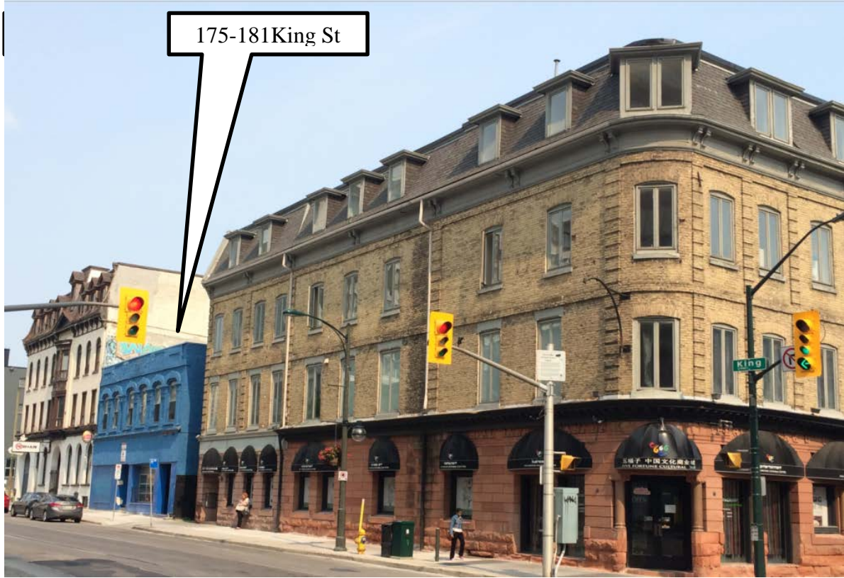
Figure 2 – 175-181 and 183 King Street Within Heritage Streetscape (looking east)
