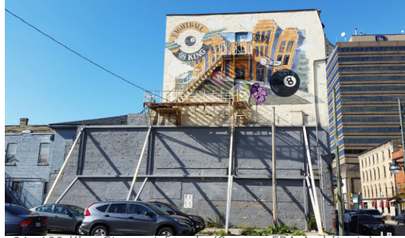
31. 183 King St., east facade (Source: ERA Architects)
