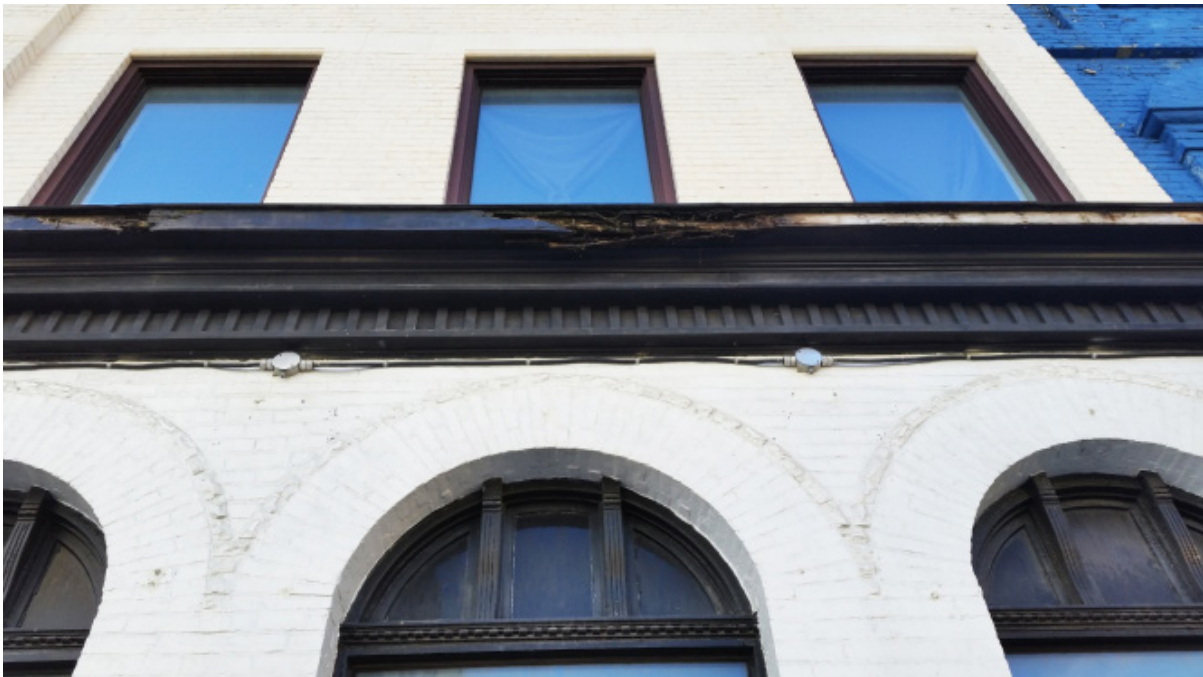
29. 183 King St., arched windows and cornice (Source: ERA Architects)
