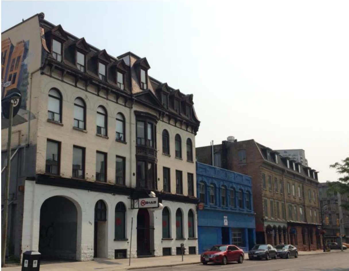
Figure 1 – 175-181 and 183 King Street Within Heritage Streetscape (looking west)
