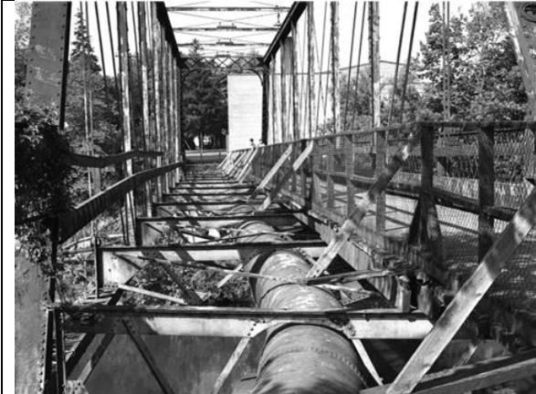
Image 5: Exposed suspender sewer of the King Street Bridge during rehabilitation work (courtesy of the *London Free Press*, 1958).
