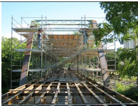
Image 8: Rehabilitation work on the King Street Bridge (courtesy of the City of London, 2010).
