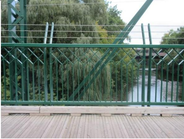
Image 11: Detail of the hand railing, installed as part of the 2010 rehabilitation program (September 29, 2015).
