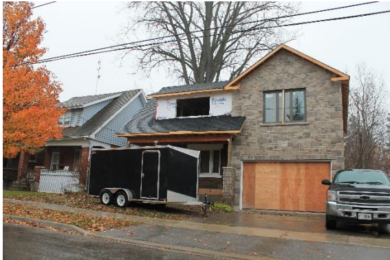
A side addition that is not compatible with the neighbourhood or the existing building in terms of scale, massing, garages, parking or materials and architectural detail.
