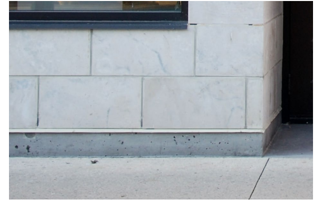
Façade materials in London, ON
