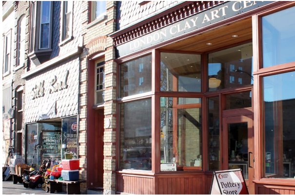
Minimized height of sign band to maximize the size of display windows, London, ON
