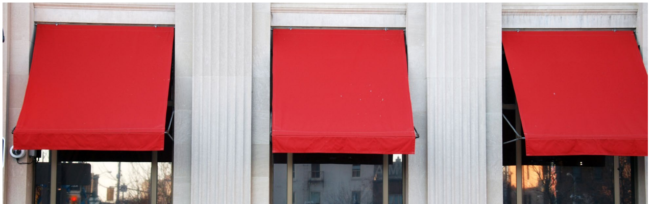
Awnings installed in Downtown London, ON
