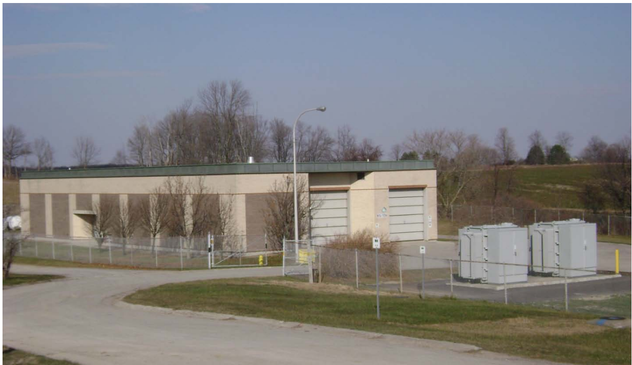
Exterior of the Arva Pumping Station
