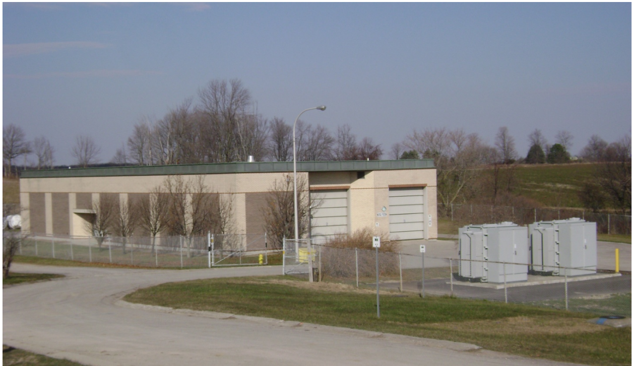
Exterior of the Arva Pumping Station
