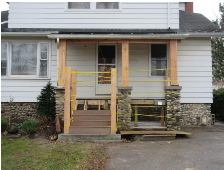
Image 3: Detail of porch at 281 Grosvenor Street (December 1, 2015).
