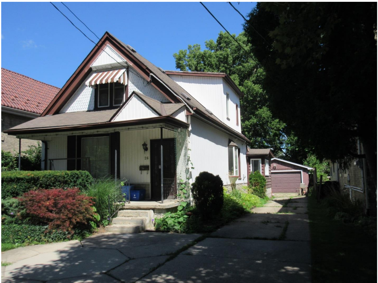
Image 2: 26 Elmwood Avenue East (August 3, 2015).
