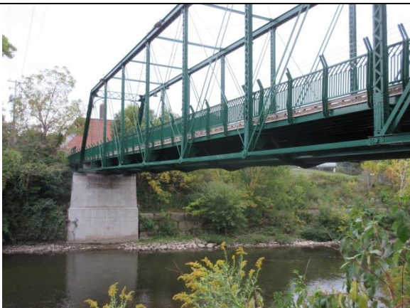
Image 15: West abutment, with suspended sewer (September 29, 2015).
