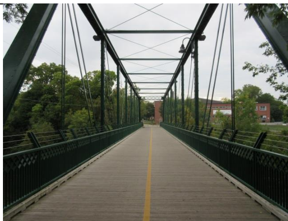
Image 10: King Street Bridge, looking west (September 28, 2015).
