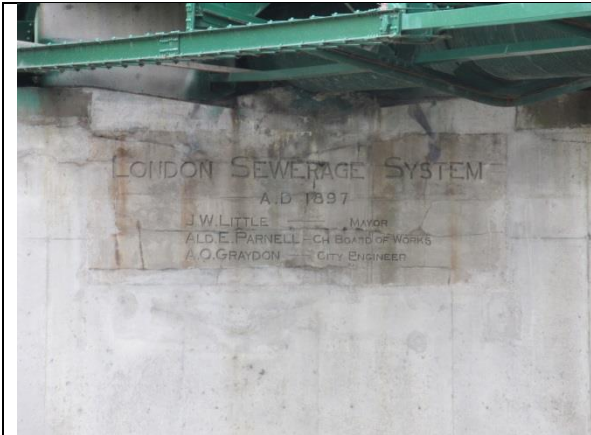
Image 17: Inscription on the west abutment of the King Street Bridge (September 29, 2015).
