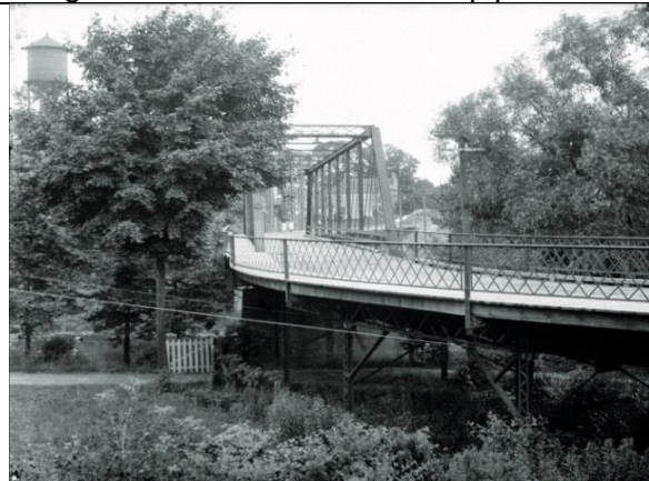
Image 3: King Street Bridge with elevated approaches, now buried (no date).
