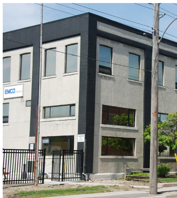
The former Reid Bros. & Co. Paper Box Manufacturing 2014.
