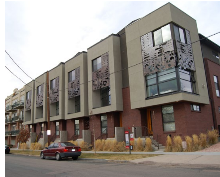
EXAMPLE: INTERESTING MATERIALS AND FACADE COMPOSITION. (TOWNHOUSE IN DENVER, COLORADO. PHOTO BY BUTTERBEAN FROM FLICKR).
