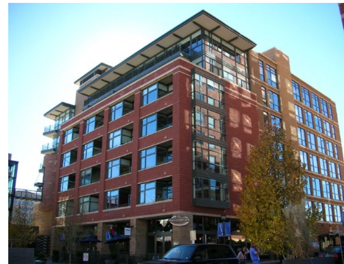
EXAMPLE: ARTICULATED BUILDING MASSING AND DIFFERENTIATION OF MATERIALS. (MIXED USE BUILDING IN DENVER, COLORADO. PHOTO BY ARCHITECTURE, FOOD & ONE LITTLE BEAUTIFUL GIRL FROM FLICKR).
