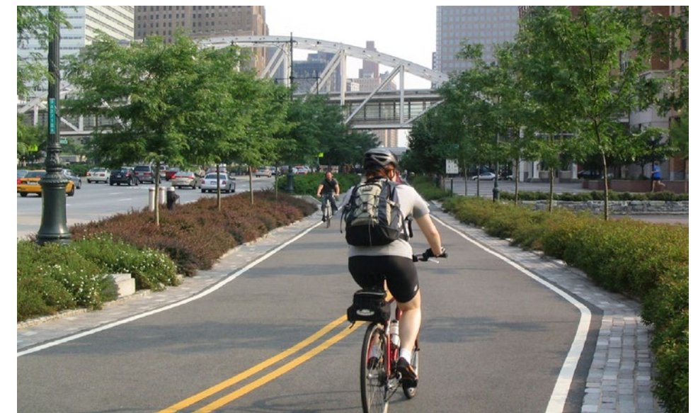
TWO LANE BIKE ROUTE SEPARATED BY GROUND-LEVEL PLANTING BEDS. (ROUTE 9A URBAN BOULEVARD, NEW YORK, NEW YORK. PHOTO BY STANTEC).
