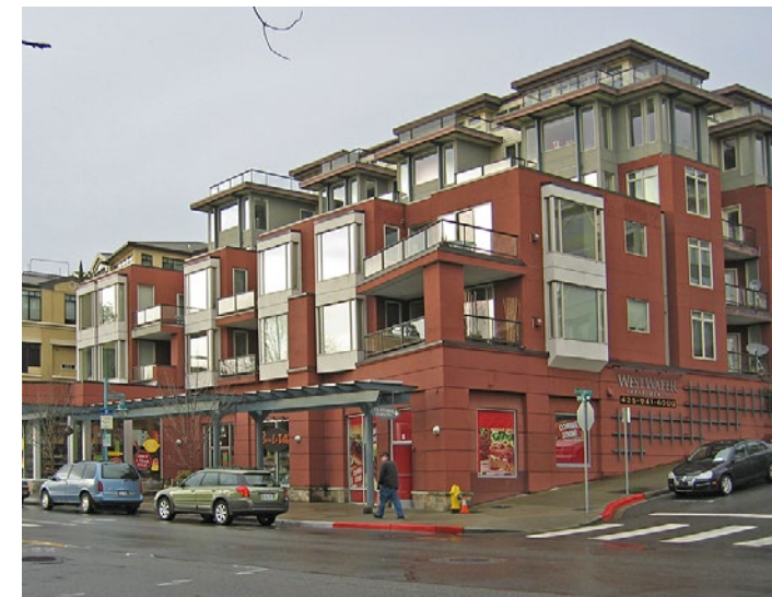
EXAMPLE: TERRACING TO CREATE OUTDOOR PATIO SPACES. (MIXED-USE INFILL DEVELOPMENT IN DOWNTOWN KIRKLAND, WASHINGTON. PHOTO BY BRETT VA FROM FLICKR).
