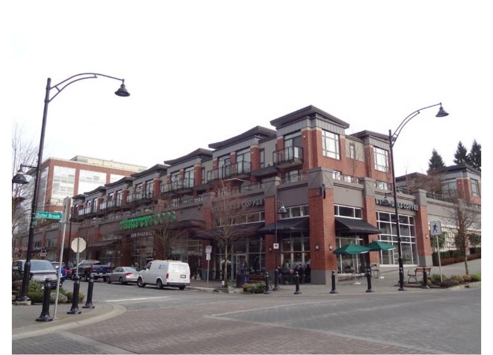
MID-RISE RESIDENTIAL DEVELOPMENT WITH GROUND RELATED RETAIL. (SUTOR BROOK IN PORT MOODY, B.C. PHOTO BY STANTEC).
