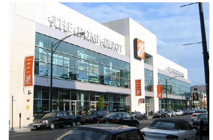
EXAMPLE: THIS HOME DEPOT HAS A NEUTRAL RETAIL FRAMEWORK AND ITS TRANSPARENCY AND SIGNAGE BANNERS ALLOW TENANT STOREFRONT EXPRESSION. (HALSTED PARK HOME DEPOT IN CHICAGO. PHOTO BY PAYTON CHUNG FROM FLICKR).
