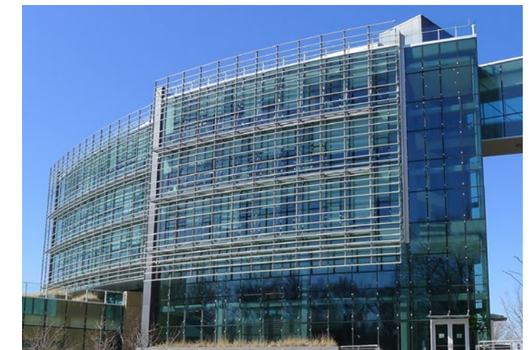
EXAMPLE: CLADDING WITH PASSIVE SOLAR SHADING. (SIMONS CENTER STONEY BROOK UNIVERSITY. PHOTO BY DANSKI14 FROM FLICKR).
