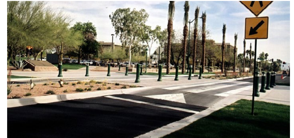
RAISED PEDESTRIAN CROSSING. (17th AVENUE, PHOENIX, ARIZONA, PHOTO BY STANTEC).
