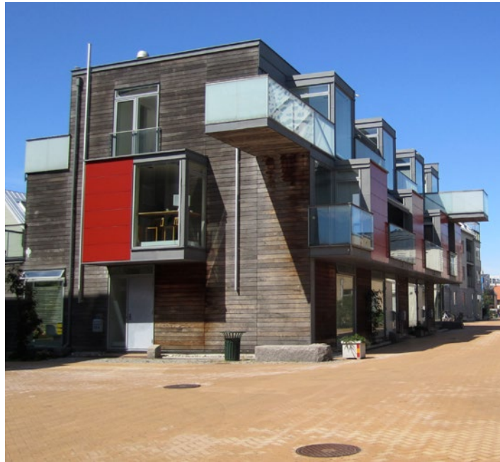
EXAMPLE: AN INTERESTING END CONDITION AND AN OPPORTUNITY FOR OUTDOOR TERRACE SPACE. (TOWNHOUSE UNITS IN STOCKHOLM, SWEDEN. PHOTO BY LA CITTA VITA FROM FLICKR).
