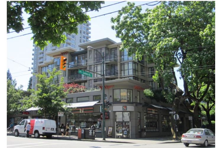
EXAMPLE: CONNECTION BETWEEN MIXED USE RESIDENTIAL & STREET RELATED RETAIL. (CONDO ON CARDERO ST. PHOTO BY LA CITTA VITA FROM FLICKR).
