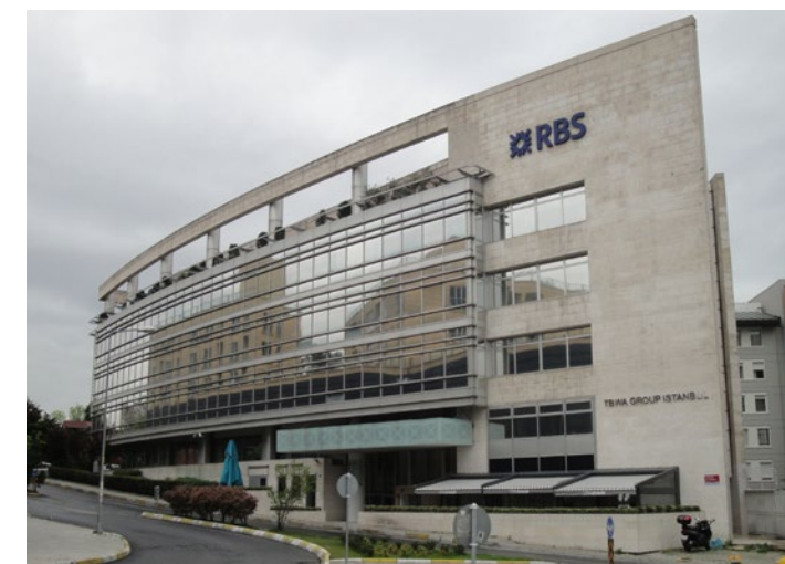
EXAMPLE: INTEGRATED & HIGH VISIBILITY SIGNAGE. (RBS HEAD OFFICE IN ISTANBUL, TURKEY. PHOTO BY REISE REISE FROM FLICKR).
