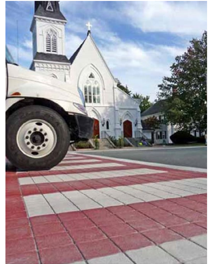
STAMPED & COLOURED ASPHALT CROSSING. (TRAFFICSCAPES - TRAFFIC PATTERNS XD).
