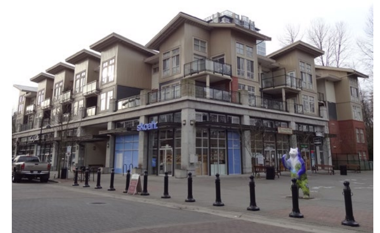
MID-RISE RESIDENTIAL DEVELOPMENT WITH PROMINENT GROUND RELATED RETAIL. (SUTOR BROOK IN PORT MOODY, B.C. PHOTO BY STANTEC).
