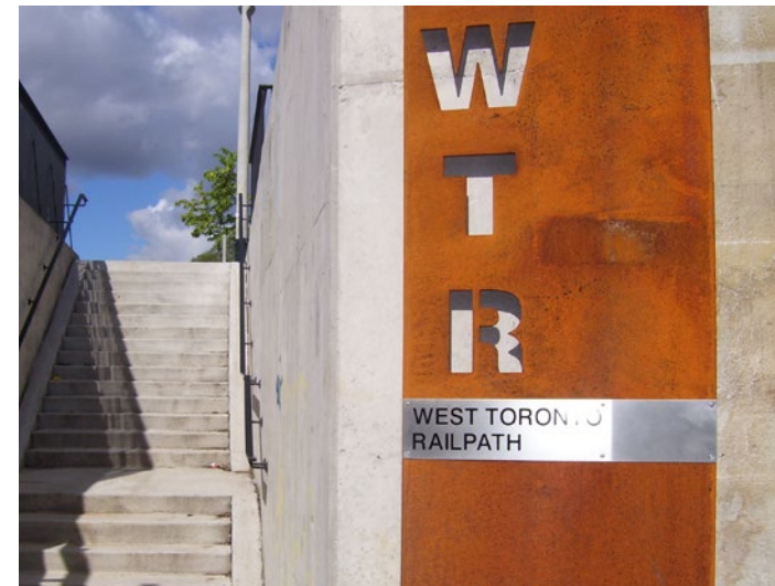
INCORPORATE SIGNAGE INTO VARIOUS ELEMENTS SUCH AS RETAINING WALLS, BRIDGES, AND PLANTERS TO ENCOURAGE WAYFINDING. THIS IS A MINIMAL BUT EFFECTIVE WAYFINDING STRATEGY. (WEST TORONTO RAIL PATH SIGNAGE. PHOTO BY STANTEC).
