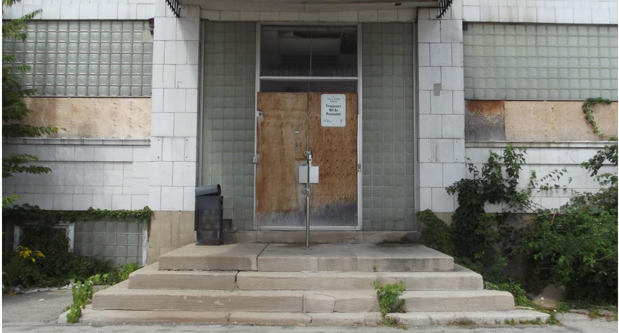
Figure 3 – Existing condition of central main entrance to original McCormick Factory building
