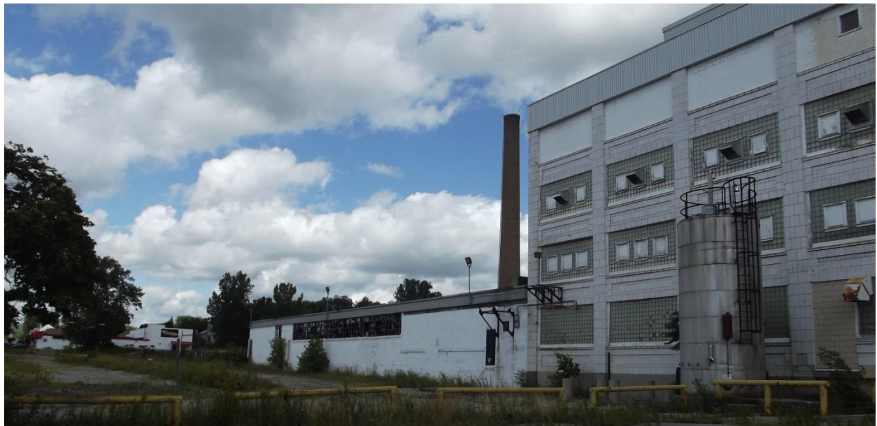
Figure 6 – Existing condition of McCormick Boulevard facing façade showing west portion of McCormick Factory (both original 4 storey front portion and 1922-1958 rear addition). The existing chimney was built sometime between 1926 and 1958, made of brick and located on the west of the former powerhouse.
