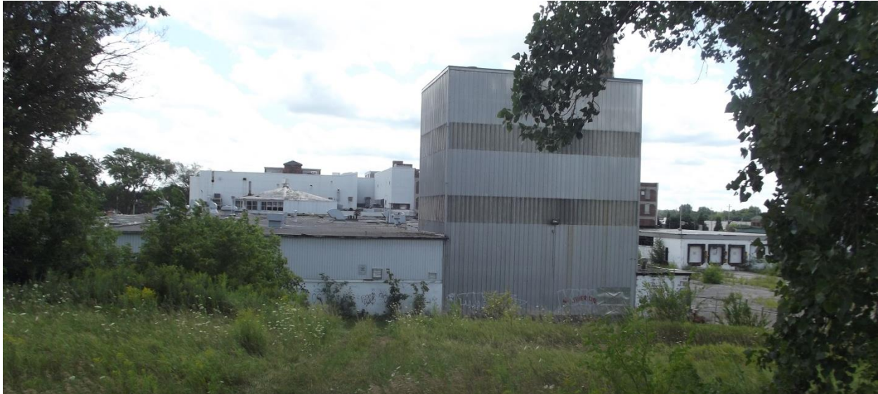
Figure 7 – Existing condition of rear portion of subject lands showing rear facing of McCormick Factory building (blending of original 1913/1914 construct and both 1922-1958 and post 1950s additions). Note the grade significant grade change from a high point on the northwest corner of the site (foreground) dropping in elevation throughout the site to both the south and east (background).
