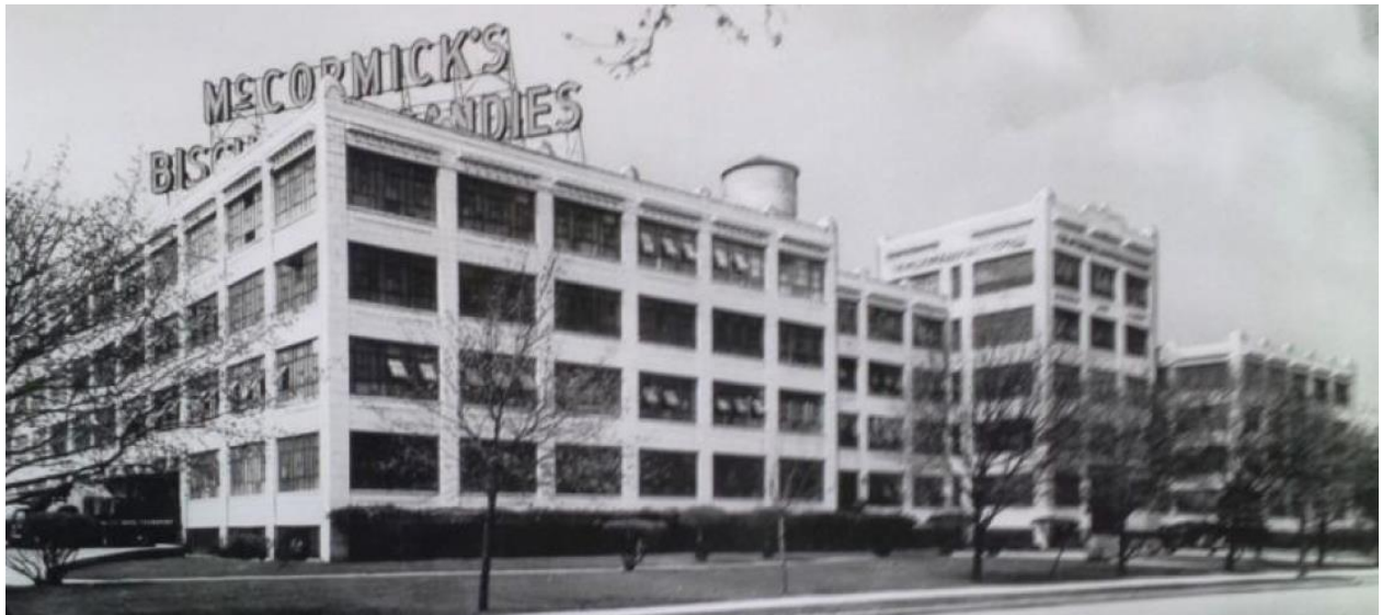
Figure 2 – Original McCormick’s Factory Building showing Dundas Street façade of five story centre block and location of decorative parapet terra cotta. (Source: June 23, 2015 Heritage Impact Assessment)
