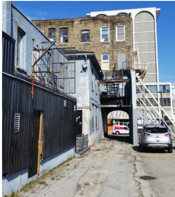
33. 183 King St., south facade and carriage way (Source: ERA Architects)
