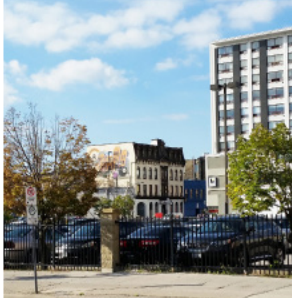
20. Contextual view from the east (Source: ERA Architects)
