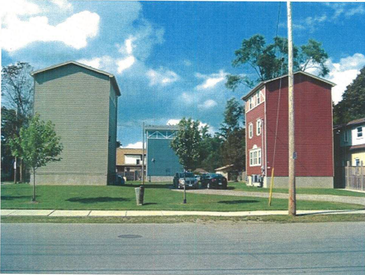
Figure 4 – Existing single detached dwellings (view facing north at the terminus of Saint George Street)
