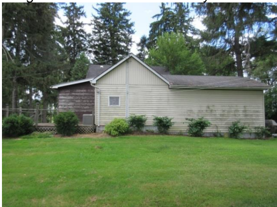
Image 7: North (rear) façade
