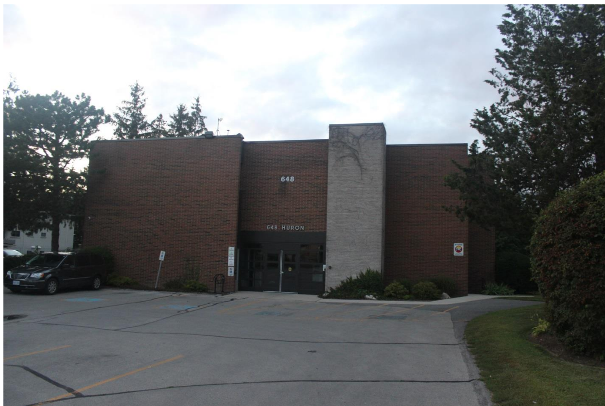
View of the existing building from Huron Street.
