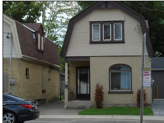
82 Oxford Street (south side)
