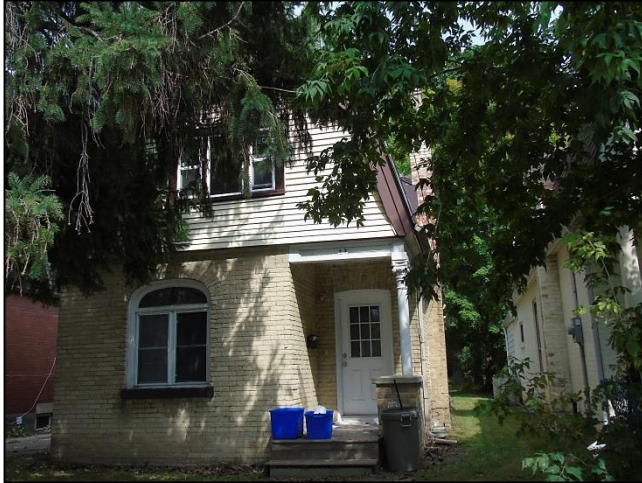
89 Oxford Street West (north side)
