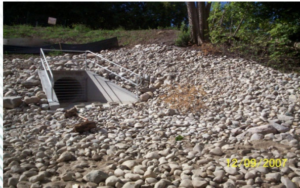
1200mm storm sewer outlet to Thames River under Ridout St. Bridge
