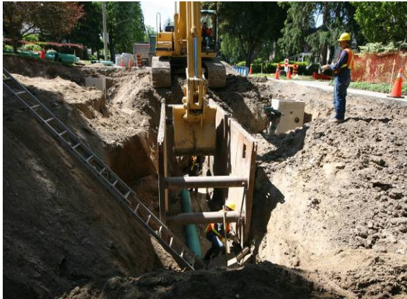
Wortley Road ~ sanitary sewer construction
