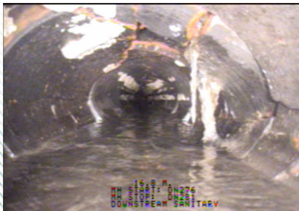
Adelaide Street ~ downstream sanitary
