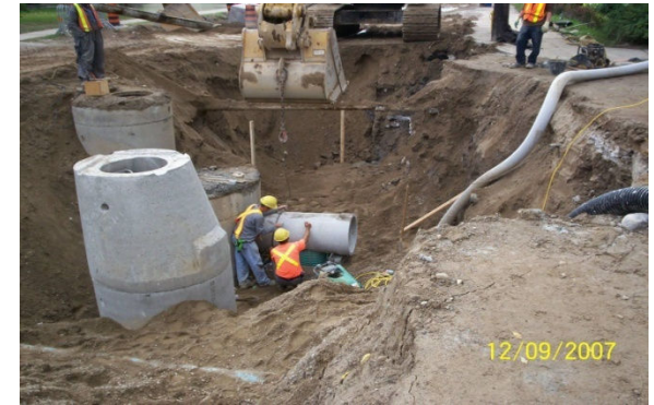
Installation of 525mm storm sewer and drop structure on Ridout St.
