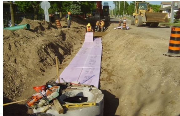
Storm sewer installation with insulation for frost protection
