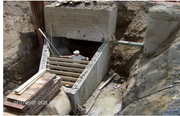
Custom Taper at existing storm manhole on Edward St.
