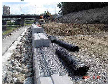
Barrier Work along Thames River
