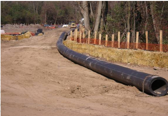
Medway Trunk Sanitary Sewer
