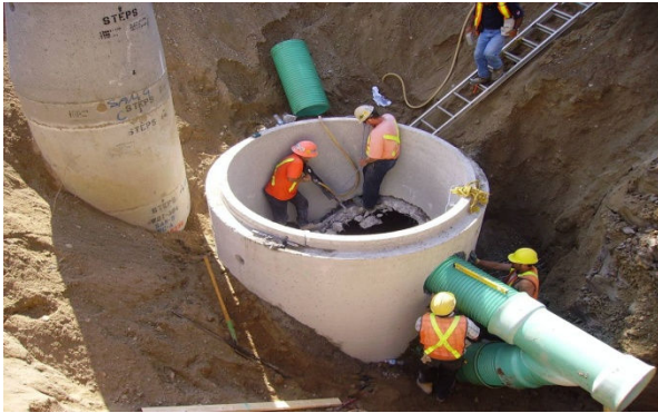
Installation of doghouse storm manhole on Belgrave
