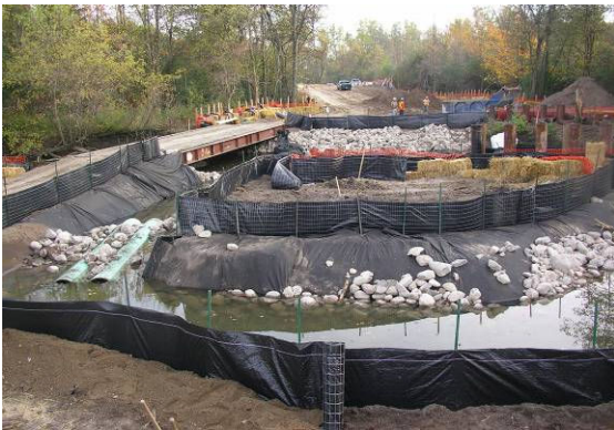
Medway Trunk Sanitary Sewer
