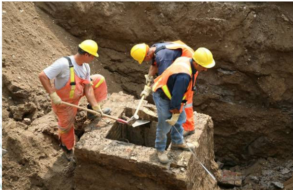
Becher Street ~ old brick manhole
