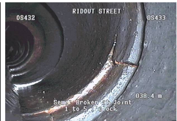
Ridout Street ~ broken at joint
