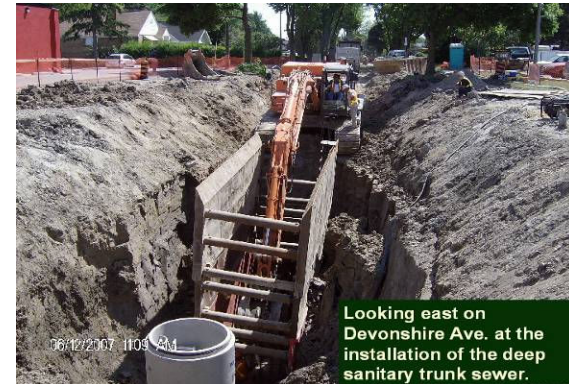
9m deep Sanitary Sewer using double trench box on Devonshire
