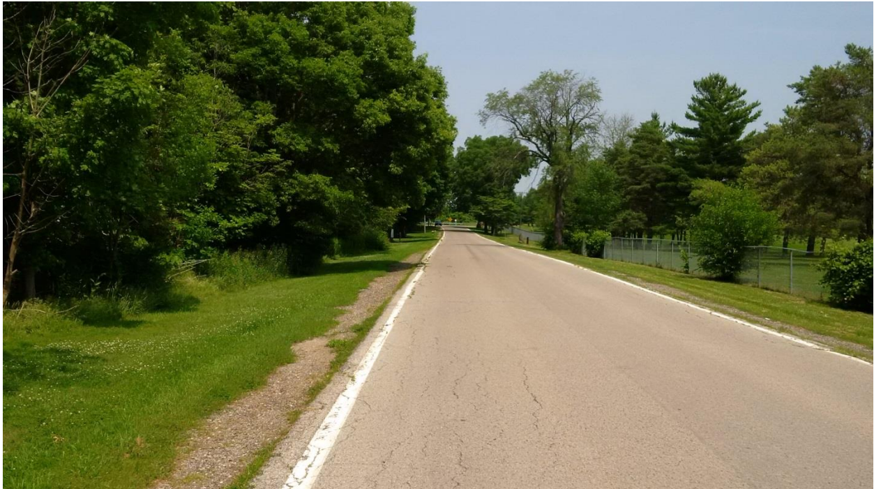
Sunningdale Road frontage, looking east
