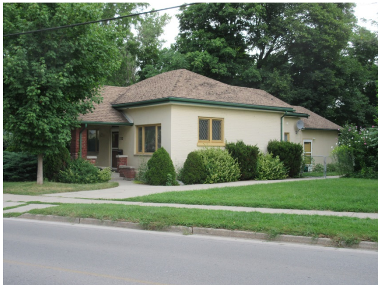
Image 2: South-west façade of 122 Wortley Road (August 10, 2015).
