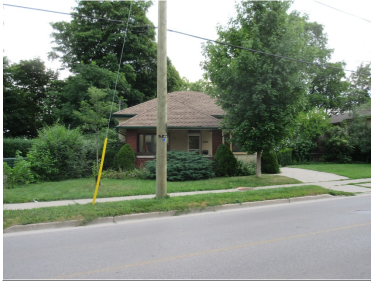
Image 1: West façade of 122 Wortley Road (August 10, 2015).
