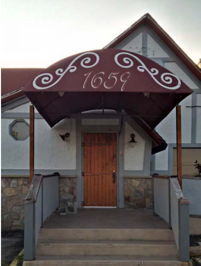
Fig. 3: Detail of front entrance property
