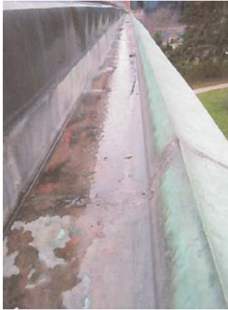
Fig 3: Copper gutter & metal flashing
