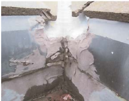
Fig 5: Transept valley at gutter
