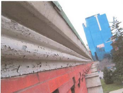
Fig 1: Cornice, galvanized metal painted
