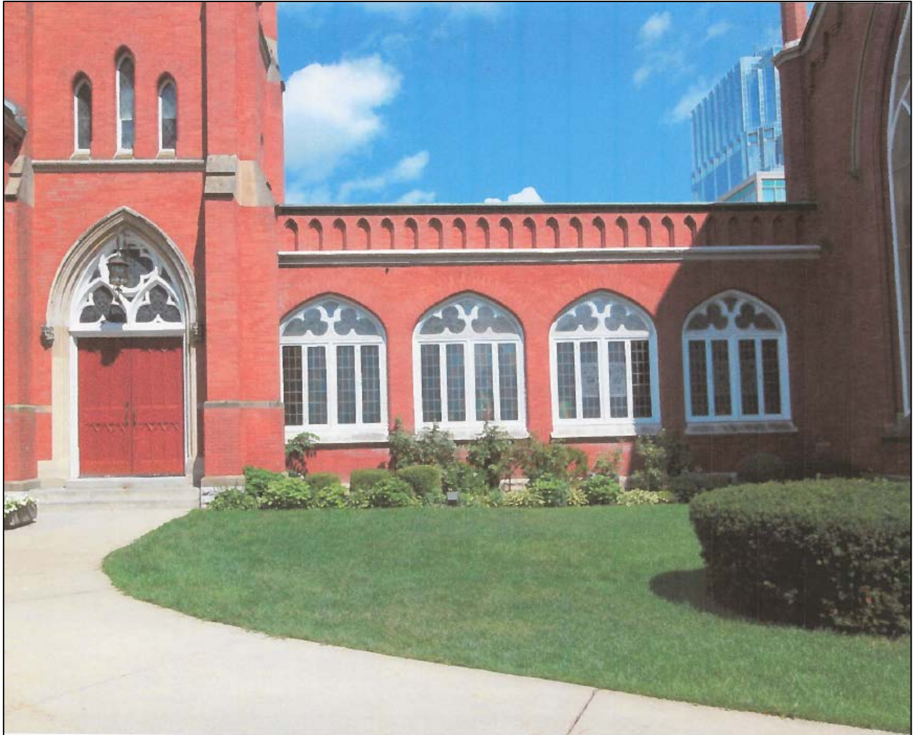
Fig 1: The west entrance of Cronyn Hall showing door elevation
