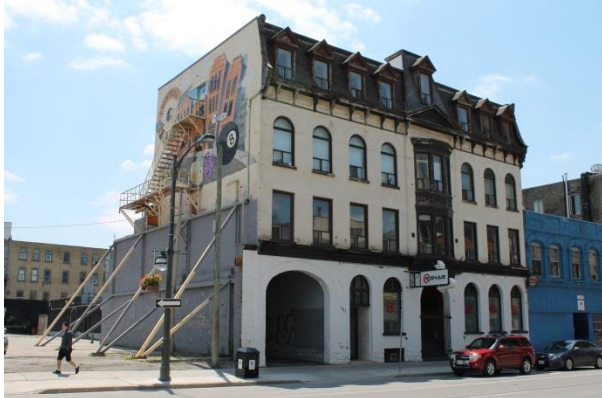
North and west facades viewed from King Street
