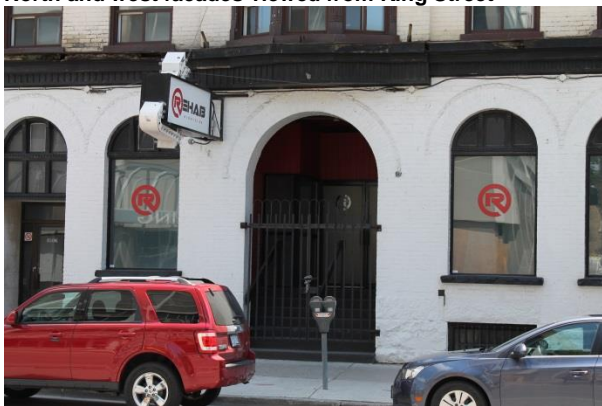
Detail - ground floor round-arch door and window openings, and recessed entrances
