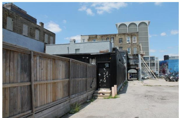
View from south showing multiple building additions above fence
