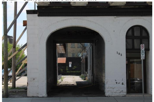
Detail - carriage-way facing King Street
