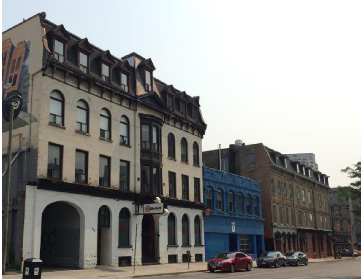
Figure 6 – 175-181 and 183 King Street Within Heritage Streetscape (looking west)
