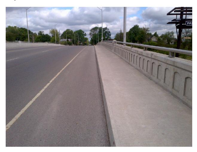
The narrowing of the road from four lanes to three and addition of wider than standard cycle lanes (1.8m) between the lanes and sidewalks has provided pedestrians with a significant buffer from vehicular traffic.
