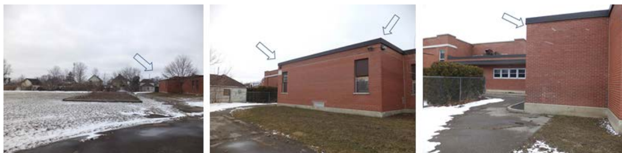
Figure 7 – Proposed Removed Portion (Southwest corner of the building)
