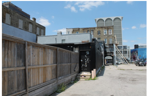
View from south showing multiple building additions above fence
