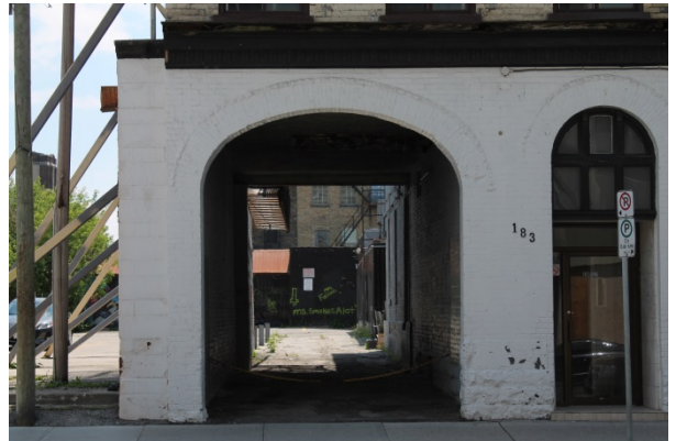
Detail – carriage-way facing King Street
