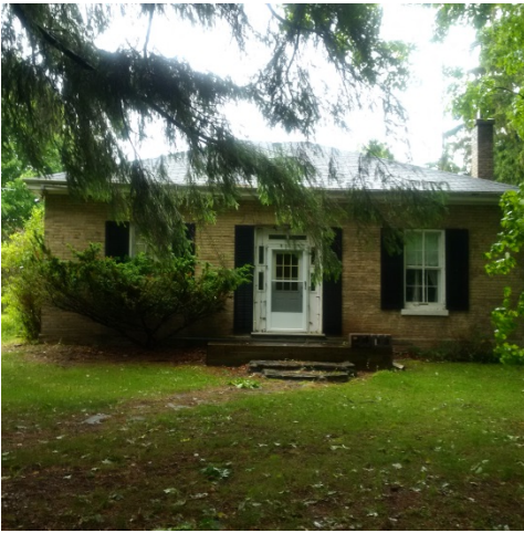
South façade facing Sunningdale
