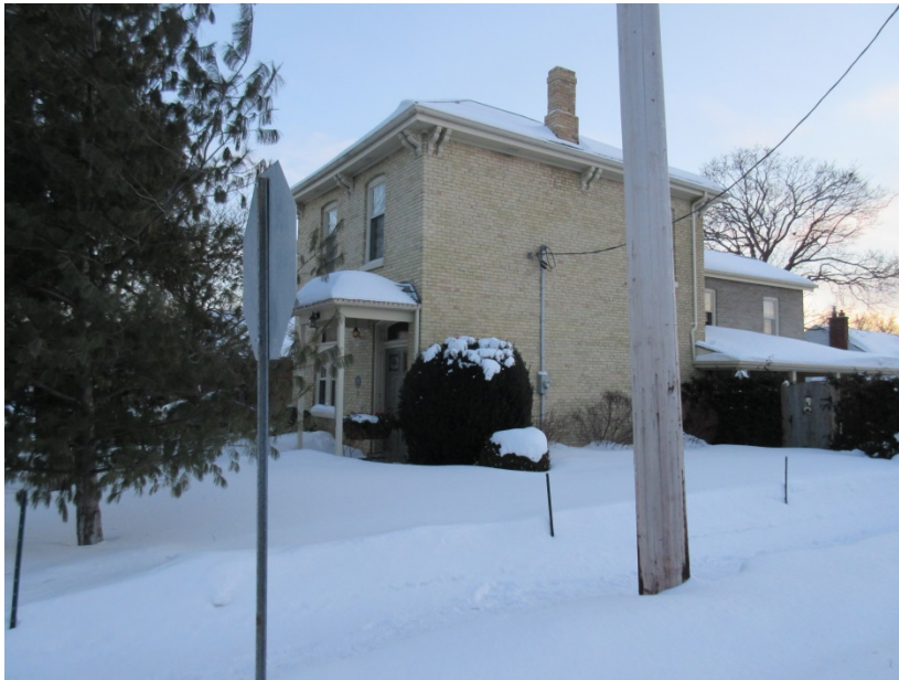
Image 2: North façade of 77 Price Street (February 25, 2015).
