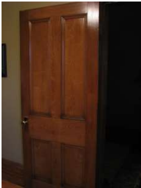
Image 9: Detail of the wood trim noted in the designating by-law (January 28, 2015) (Image courtesy of the property owners).
