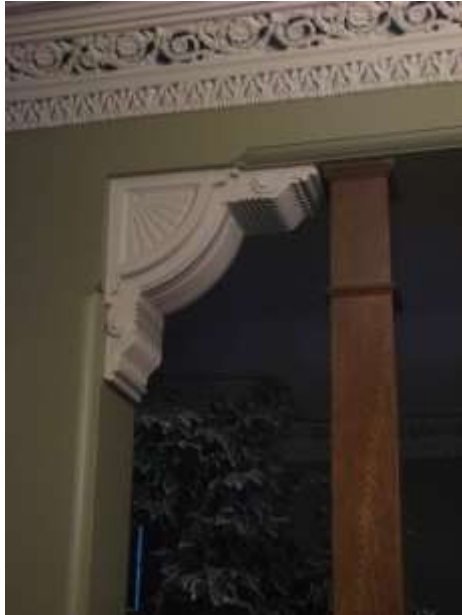
Image 8: Detail of the ornamental plaster work at 77 Price Street (January 28, 2015) (Image courtesy of the property owners).
