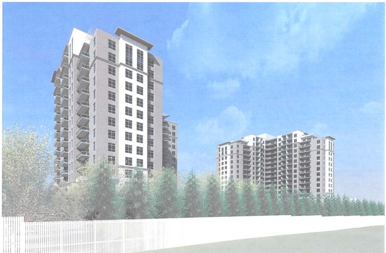
South West View
