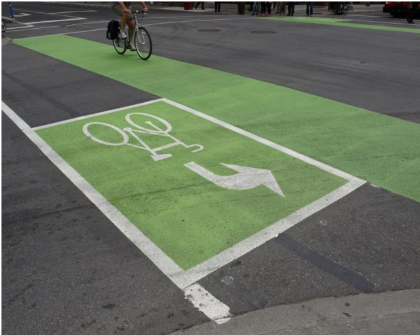
Left turn queue box and intersection pavement markings on the Laurier Bikeway in Ottawa.
