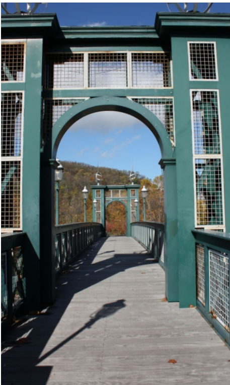
An example of a pedestrian bridge.
