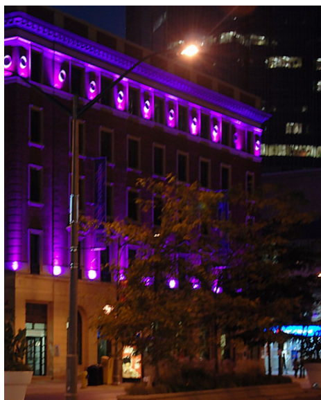
Innovative building lighting downtown.
