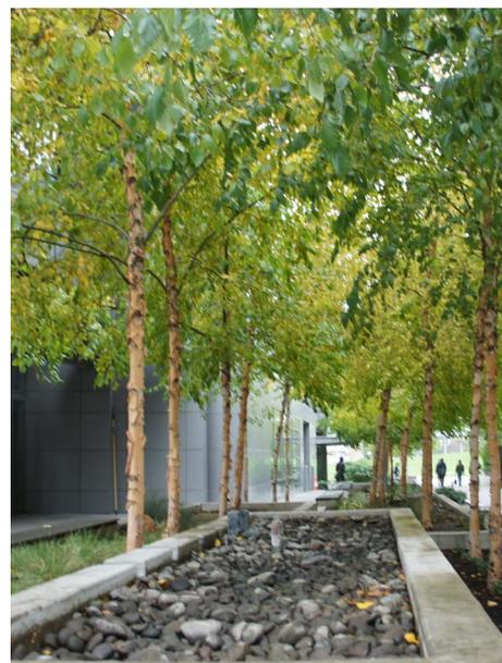
Examples of alternative stormwater management systems that slow the rainwater intake into the system, relieving pressure from the system during large storm events.
