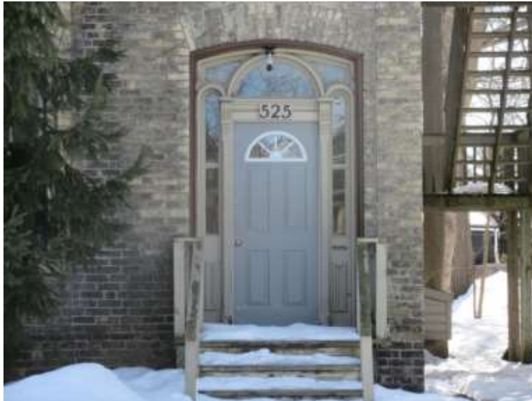
Image 4: Detail of the London Doorway at 525 Princess Avenue (March 12, 2015).
