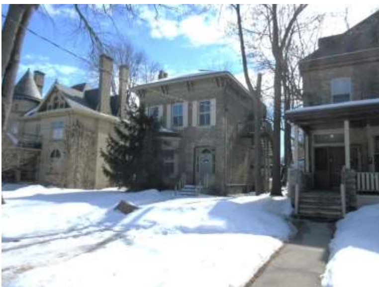
Image 3: North and west façades of 525 Princess Avenue (March 12, 2015).
