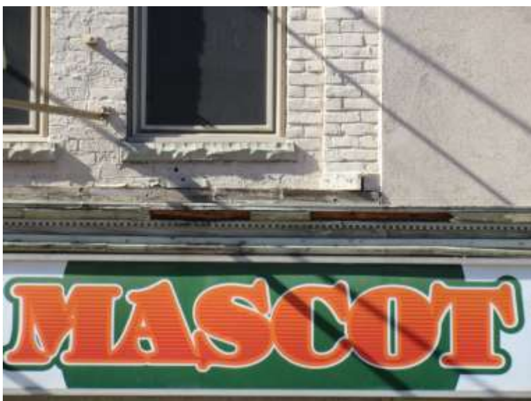
Image 3: Existing cornice at 172-174 Dundas Street (March 30, 2015).
