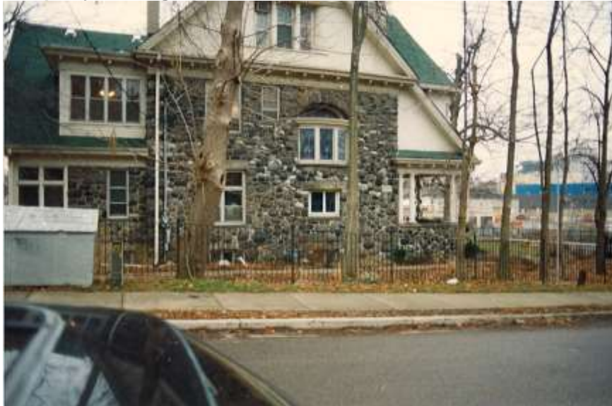
Image 1: South façade of 37 Ridout Street South. Note the large, un-coursed rubble stone construction, steeply pitched gable roof, columns on the verandah, and windows (Source: City of London files) (undated photograph).
