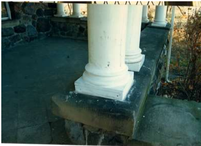
Image 2: Detail of the paired and triple columns on the verandah of 37 Ridout Street South. Note the large, un-coursed rubble stone balustrade of the verandah (Source: City of London files) (undated photograph).
