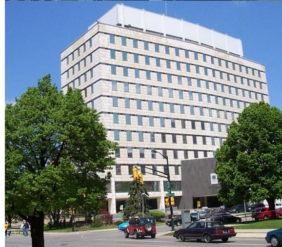
Philip Carter Johnson (architect) and Ellis Don (builder), City Hall, 1971
