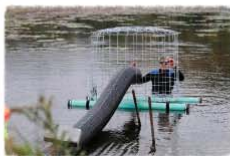
Beaver Device Installation
