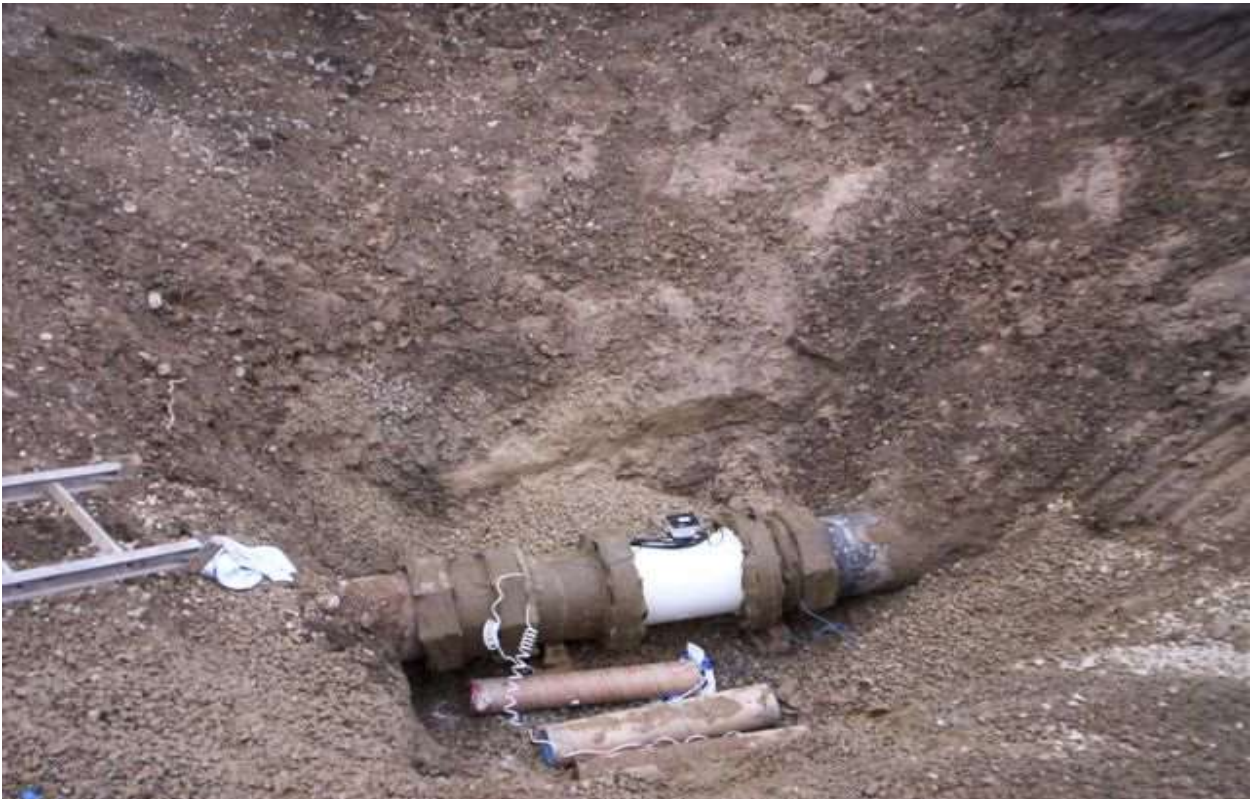
Figure 5: Electromagnetic Flow Meter Install
